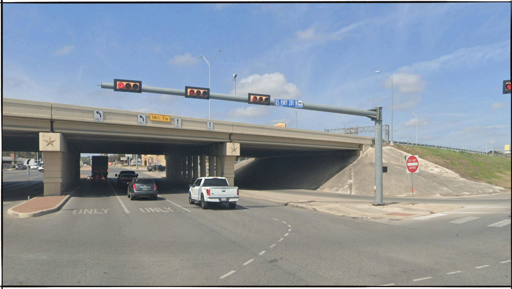
Figure 32: West Bitters Road at Hwy 281 – Existing
