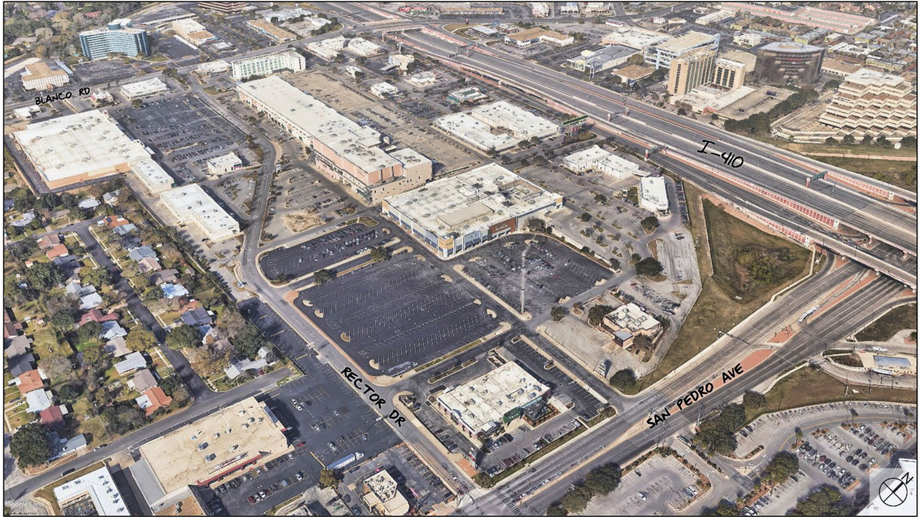
Figure 15: Transformative Project: Park North Shopping Center – Existing (looking northwest)
